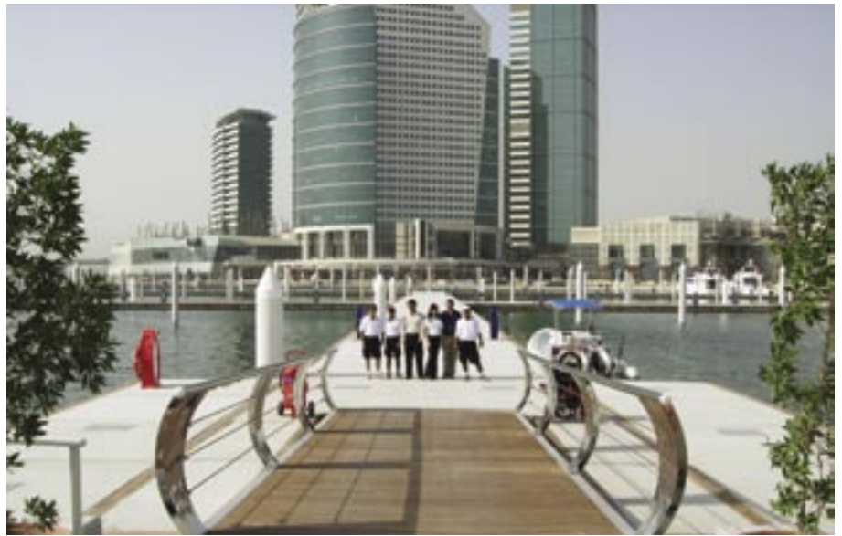
An oversized bollard in use (left) and the new-style hinged bridge with slender handrails.
